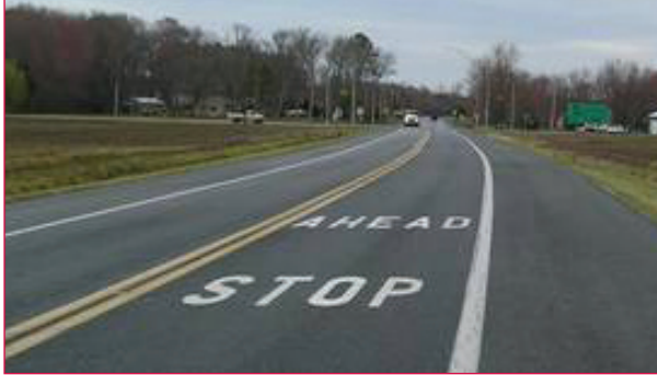
Figure 1. Example of a Rural STOP AHEAD Installation.
