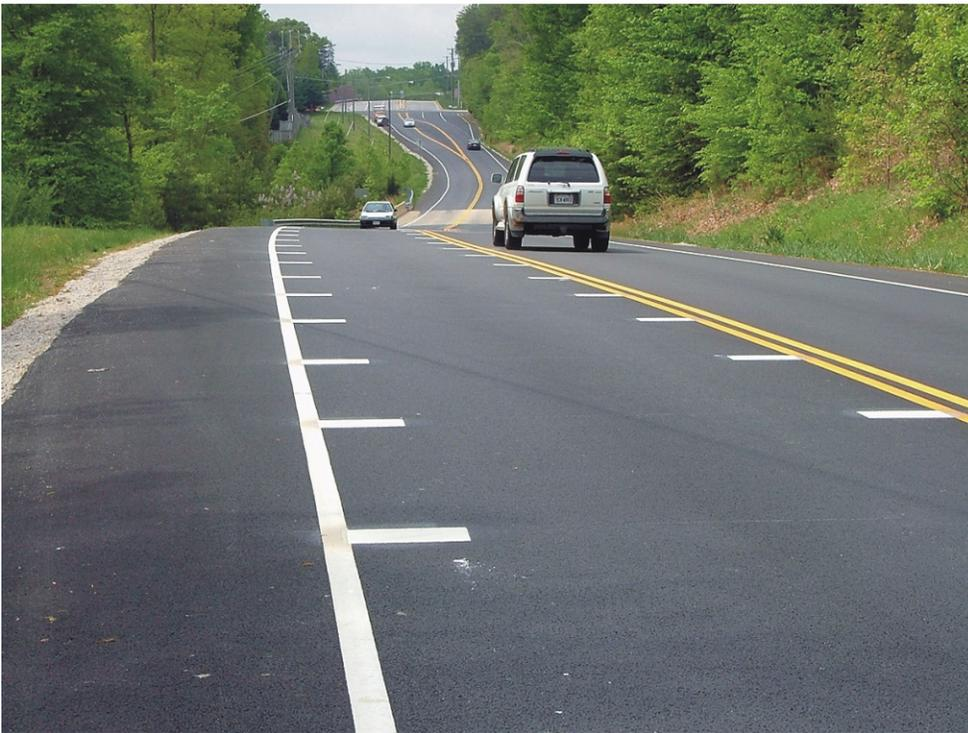
**Figure 3. Optical Speed Bars on South End of Lee Chapel Road Installation. *Top:* View Looking North. *Bottom:* View Looking South.**
