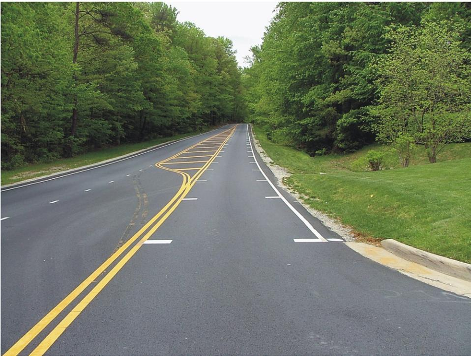
**Figure 4. Optical Speed Bars on North End of Lee Chapel Road Installation. *Top:* View Looking North. *Bottom:* View Looking South.**
