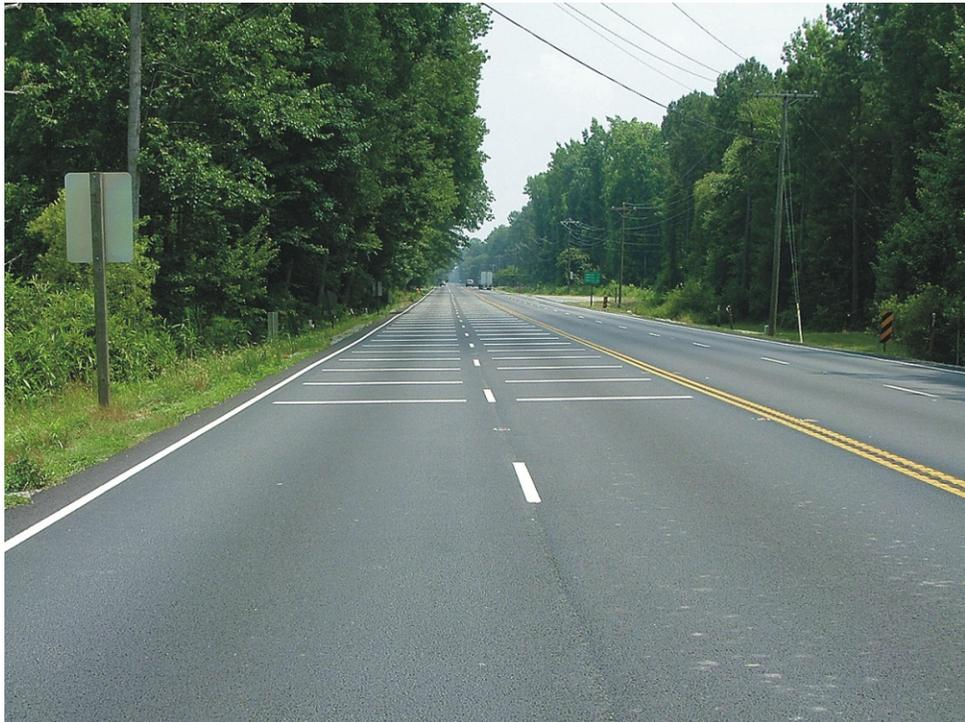
**Figure 6. Optical Speed Bars on Route 460, East Side of Zuni. *Top*, View Looking West. *Bottom*, View Looking East.**
