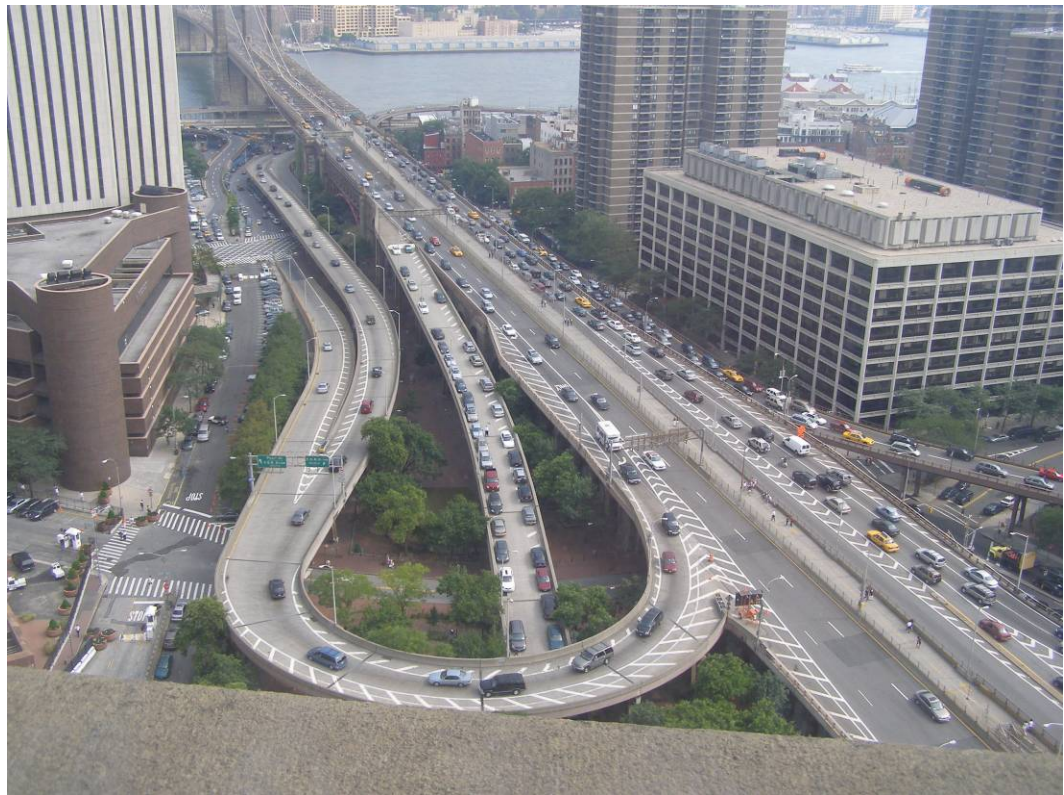
Figure 45 - Aerial Image of Law Enforcement Parking on the closed Brooklyn Bridge ramp
